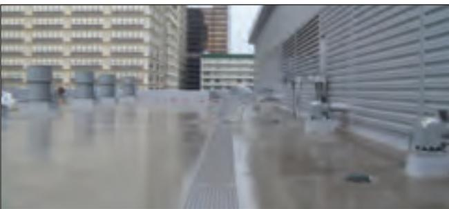
*Roof of the main lobby, located on the south end of the building. The roof was structurally sloped. Roofers installed DensDeck, two layers of ISO, saddles and mechanically fastened TPO for the roof.*
