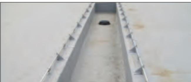
*The drainage on the main “wave” roof was provided through these large gutter bays. The Alpine snow rails were installed to break up sliding ice and prevent damage to the roofing membrane that lines the gutters.*
