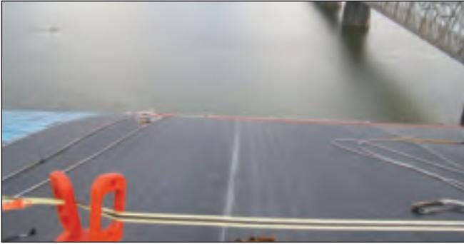
*The north side of the KFC Yum! Center is known as the “waterfall.” A Carlisle mechanically fastened system was used as an underlayment for the metal panel system that would be the finished look.*
