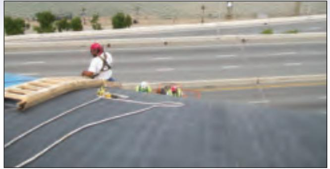
*Work was done on the waterfall using proper safety equipment and chicken ladders. When the slope became too steep, a 135’ aerial lift was used. Pictured is Laymond Daily working on a seam and Tom Tweedlie and Barry Cast positioning the lift.*
